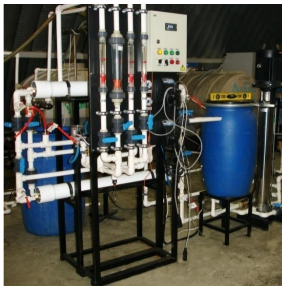
Figure 2. General view of the RO pilot installation
